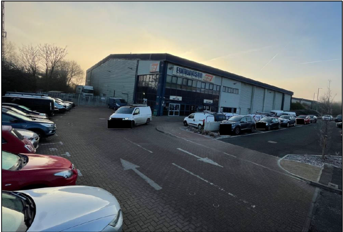
Plate 3: Image of EEL Access and Area Covered by DCO Application Order Limits
