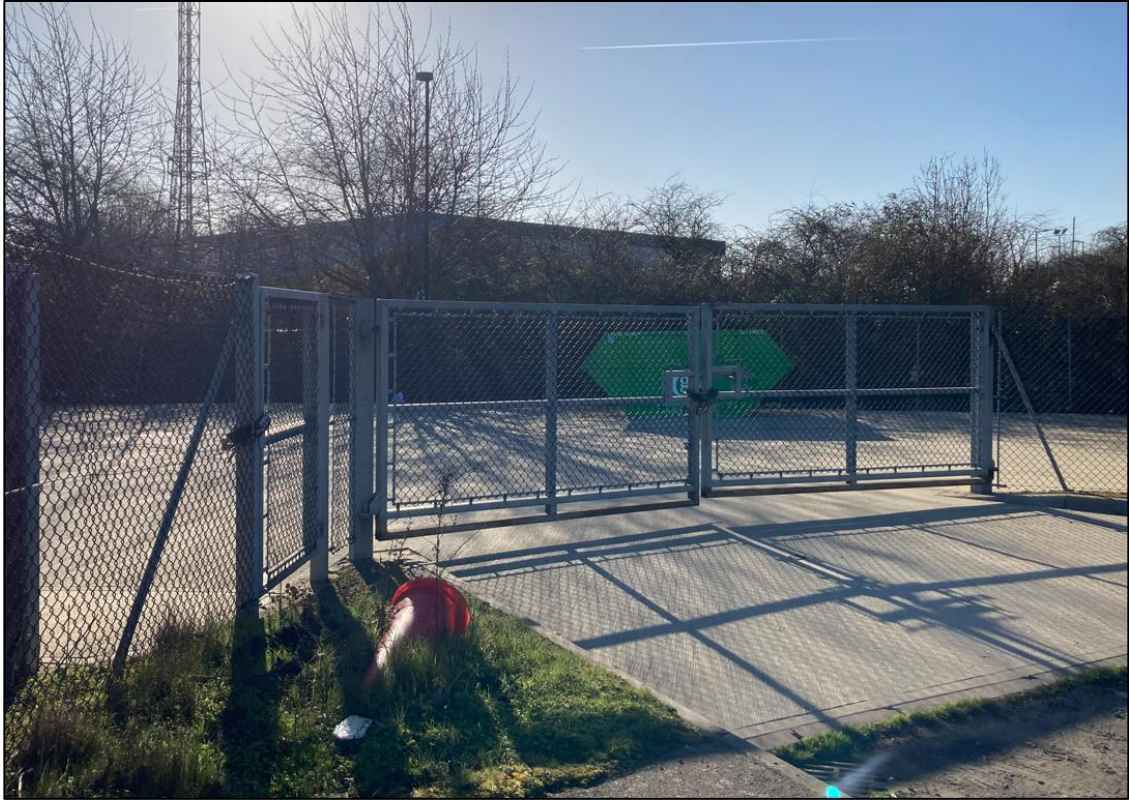
Plate 6: Trilux Lighting Service Yard Access
